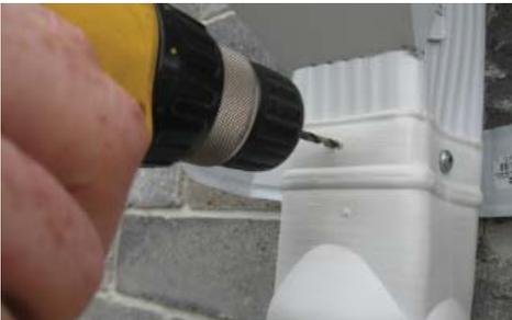
16. Place the square end of the flexible downspout in place and using a 1/8" drill bit and the provided hardware, attach the flexible downspout to the leaf catcher. Use two screws at this connection.
