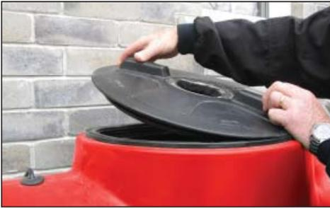
13. Place the access cover / lid in place and lock into position.
