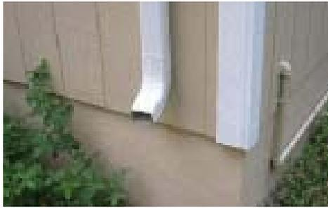
5. A location should be selected close to an existing downspout and relatively close to the house to prevent obstruction and ease of installation. Be aware of the dimension of each tank, and ensure that there is more than enough space for the tank to be permanently placed into that location.
