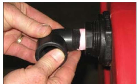
12. The other bulkhead at the top edge of the tank in used for the overflow. Attach the overflow elbow and hand tighten. A hose can be attached to redirect water overflow.
