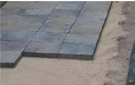
7. The best solution for placing the tank is to have a solid base which can be made of large patio stones / walkway stones or to pour a concrete base. Lay the stones into place providing enough area for the footing of the tank.
