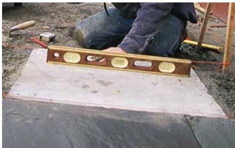
8. Level the stones to ensure that the tank sits flat and does not tilt and risk tipping. Adjust as required. Check for final level and place the tank in position.
