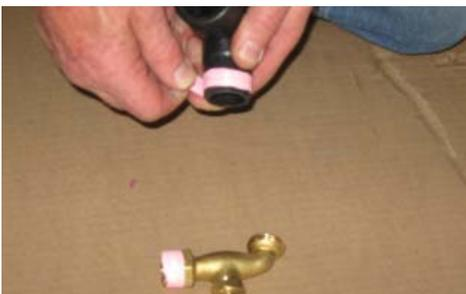
10. Using the provided roll of teflon tape, wrap 2 layers of tape on threads of the spigot and the overflow elbow to ensure proper installation and seals.
