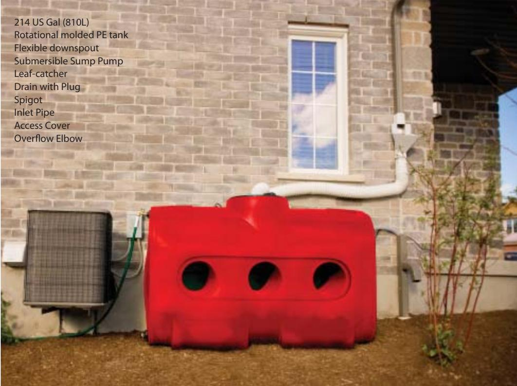
RTS Rainwater Collecting System provides an efficient, economical and unique way to store rainwater.
