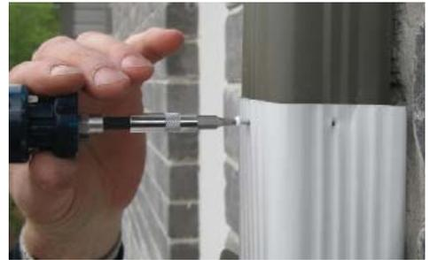
15. Using the provided screws attach the leaf catcher to the downspout. Use two screws at this connection.
