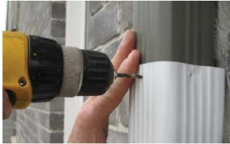
14. Locate the existing downspout that you will be using and remove sections of the downspout so that the remaining pipe is at least 1ft. higher than the top of the tank. Place the leaf catcher in position with the grate facing up, and using a 1/8" drill bit, drill through the leaf catcher and the downspout.
