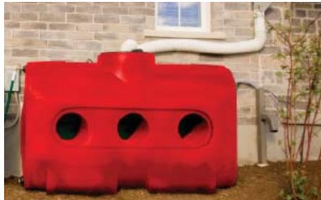
17. Attach a hose to the spigot if desired and plug the pump electrical chord into a GFI outlet for operation.
