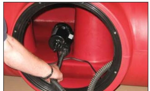
3. Place the pump back into the tank as shown. Ensure that the flexible hose is completely inside the tank.
