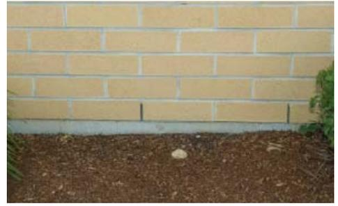
6. Clear the location from obstructions and even out the area with a spade, shovel or rake, depending on the existing surface. The ground below the tank must be level to prevent the tank from slopping. It is suggested the grade be slightly tilting in towards the building so that the tank leans just slightly towards the building and not away from it.
